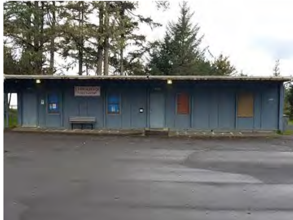
Image 70: Structure 3 - East Elevation (plywood siding with battens)
